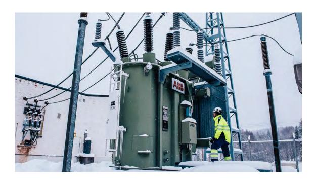
High-voltage systems may give life-threatening **electrical shocks even without direct contact**, because electrical current can pass through a gap in the air (arc). The risk of electrical shocks and arcing exists in the vicinity of electrical cables or other uninsulated live equipment and their parts. The required protection and allowed safe working distances are specified in safety plan and during local induction training.
